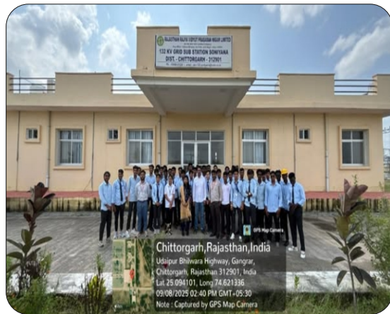
132 kV Grid Substation, Soniyana (RVPNL) Department of Electrical Engineering
