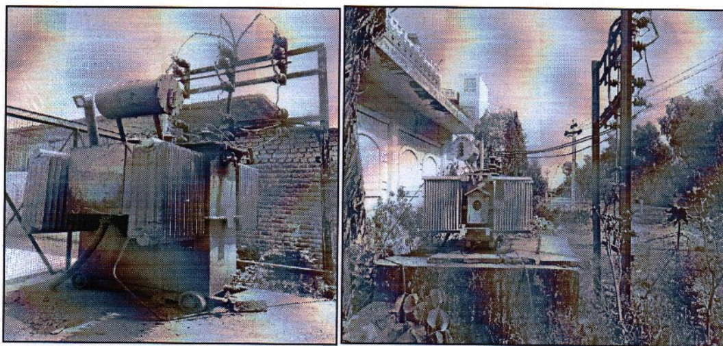
Figure 3.1:- 11 kV Feeder and 630 kVA and 500 kVA
